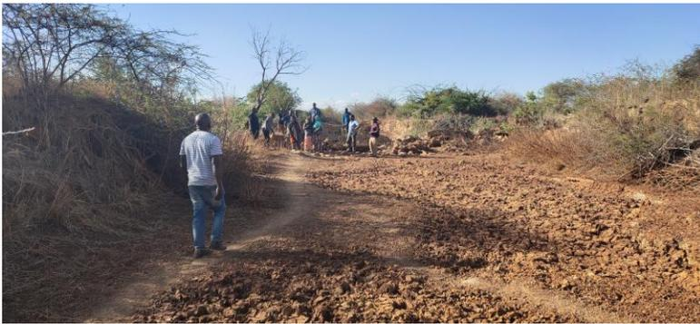
**Annex Figure 7 Broken embankment and spillway of the dam at Mtitaa causing low water storage capacity of the dam.**
