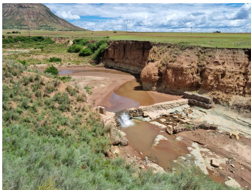
Figure 11 A sand dam constructed with IACOV support
