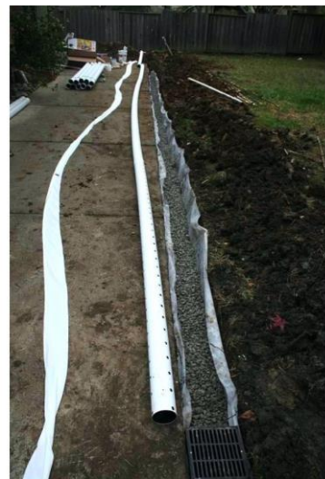
Figure 16: Technical design of proposed interventions in Khoroo 7 and 9 - Perforated pipes will be used and installed to a depth of 1m. The construction will be similar to the 'open' drainage channels and will involve land excavation, drainage pipe transportation and installation and filling with excavated soil and / or gravel. The drainage pipes selected will be of length(s) which are suitable for easy transportation and installation within an average plot size (500m 2 ) so it can be assembled on a plot by plot basis without much disturbance to neighbouring areas.
