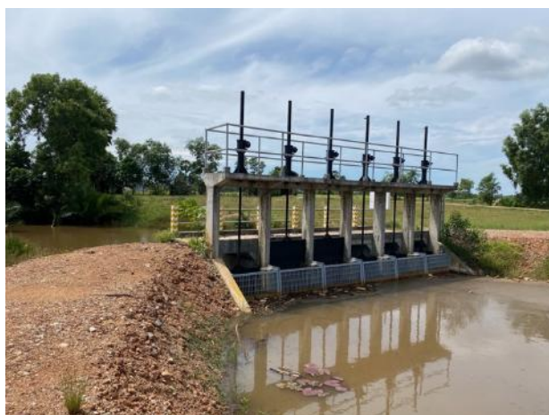
Water gate and embankments constructed in Angkaol Commune, Output 3.3 (Laura Hammett)
