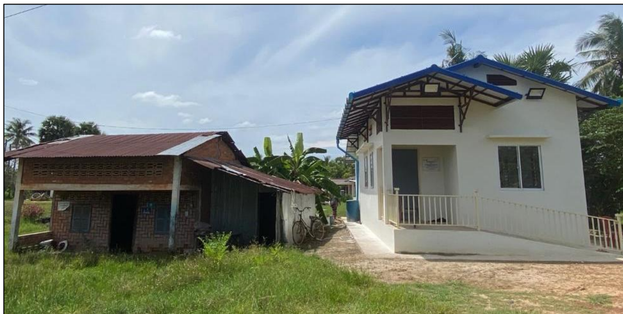
An example of the resilient houses constructed under Output 3.5 (R) with the homeowner's prior home visible to the left. (Photo: Laura Hammett)
