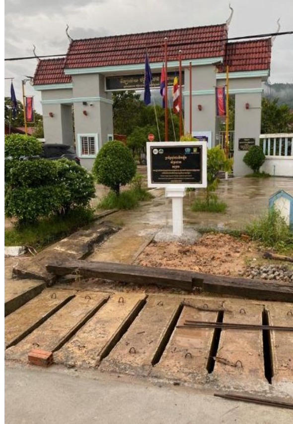
L: Construction in final stages for the pavement adjacent to the drainage channel in Veal Rinh. R: Drainage built via the project in front of Veal Rinh High School (Photos: Laura Hammett)
