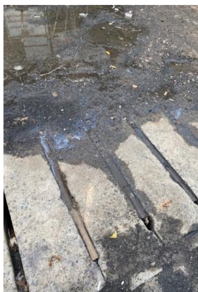
Drainage developed under the project viewed in October 2025 near the Veal Rinh Market, with silt compromising ability for water to drain. (Photo: Laura Hammett)
