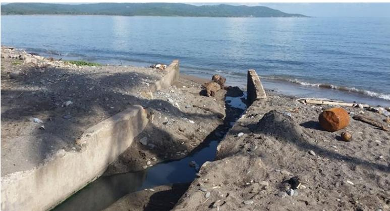
**Figure D: Motherford Drain backed up at outfall to the sea**
