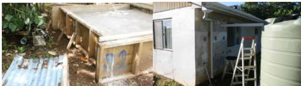
Figure 5. Installing a rainwater harvesting system at the household level (Source, PACC Niue, 2014)
