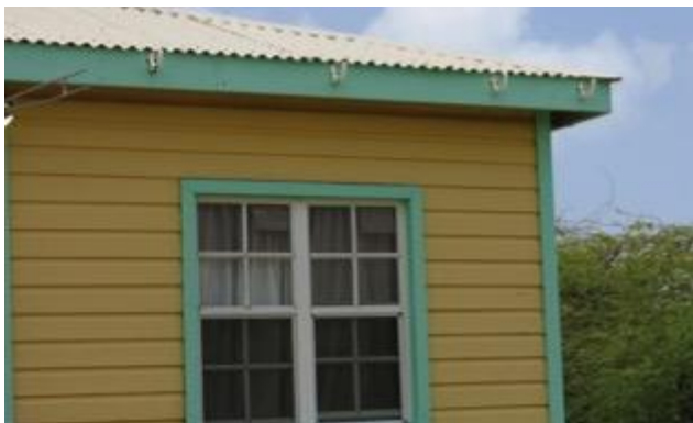
Figure 7. A household in McKinnon’s pond area with braces for rainwater harvesting but no guttering (toilets, sinks, shower heads, installed
