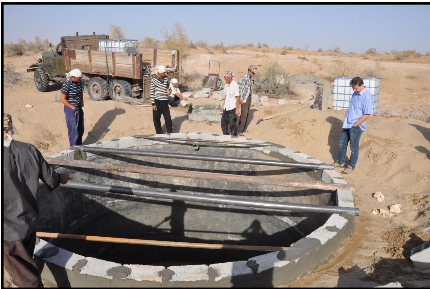
Photo: Project-supported construction of a sardob, a traditional water storage pit for collecting surface run-off from the nearby natural Takyr depression, in the Yerbent Region of the Karakum desert.
