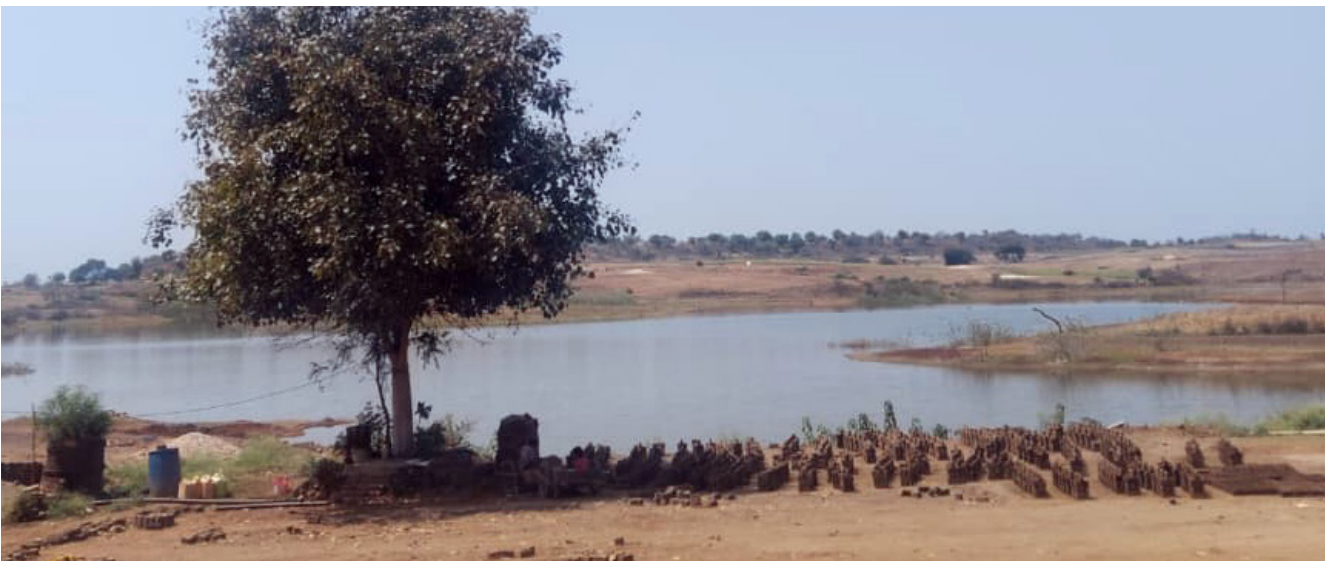
Field bunding & pond clearing
