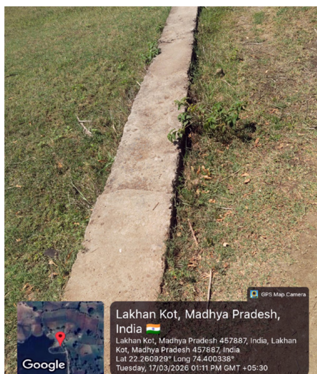
FTL (wall construction), soil and rock bunding
