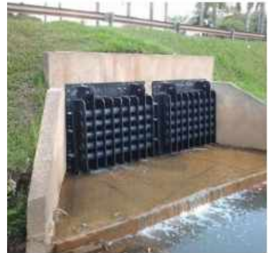
Figure 2 – Example of Flap Gate - FLOGATE HDPE, link
