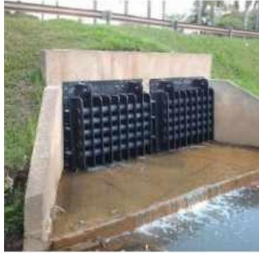
Figure 2 – Example of Flap Gate - FLOGATE HDPE, [link](#)
