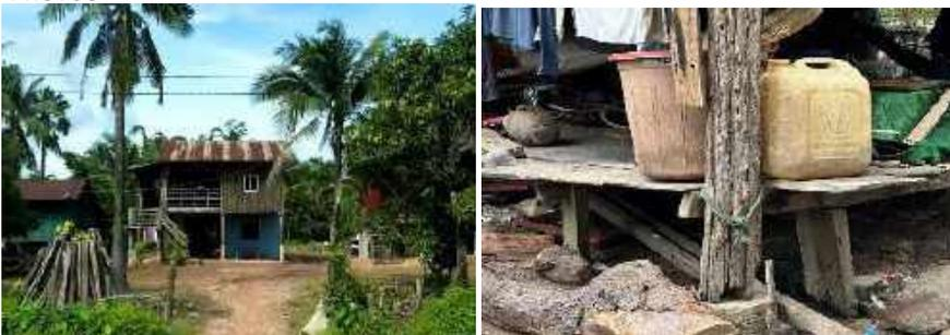
Figure 10 Typical house built on stilts design in Cambodia
