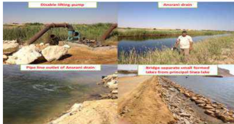
Figure 6: Water Drainage and stagnation issues
