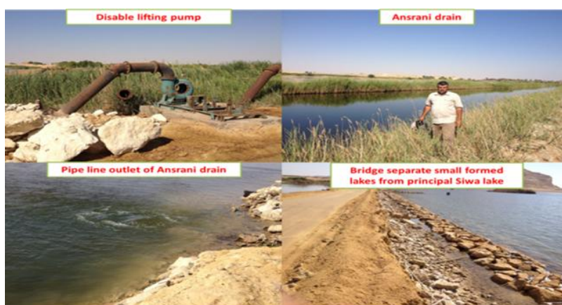
Figure 6: Water Drainage and stagnation issues
