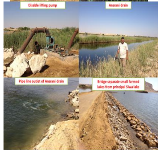
Huge quantities of drainage water
