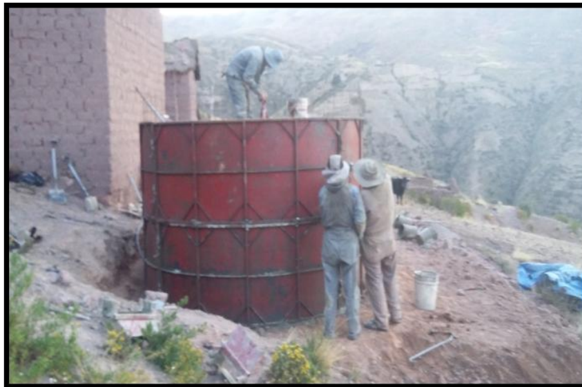
Photo 7. Concrete storage tank require a special mold with a tailored design to this technology, the programme proposes creating its own molds for the sustainability of the project
