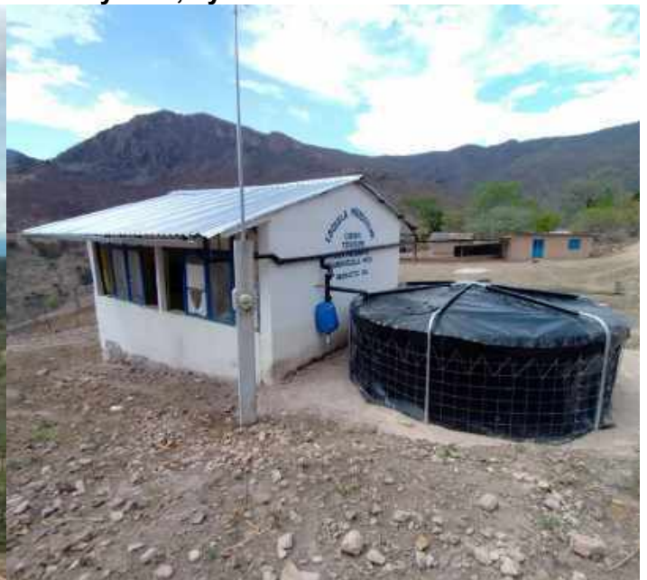
RWH system in preschool in Huamuchilillo
