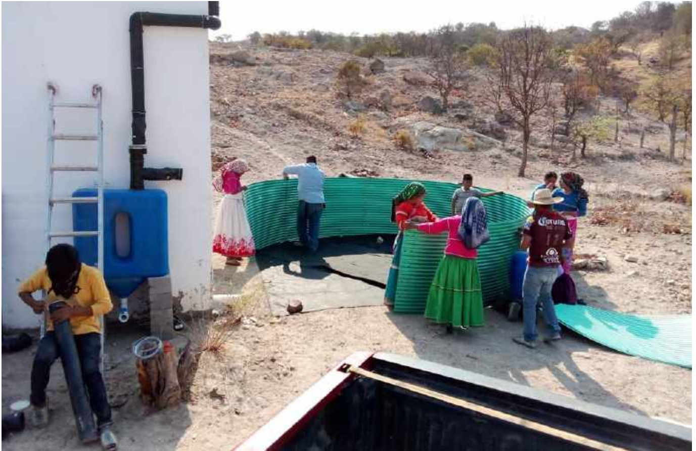
Participative cistern installation
