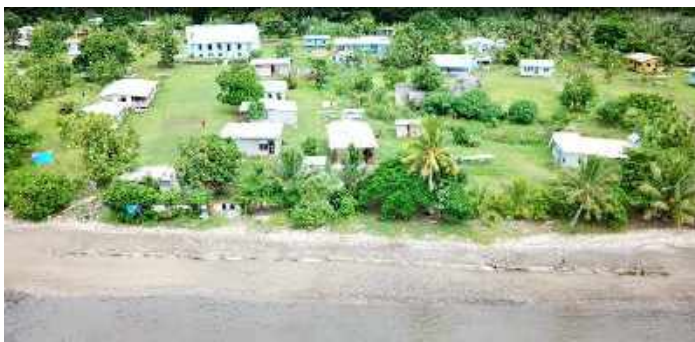
Figure 45 Site for NbS seawall installation in Nabuna Village
