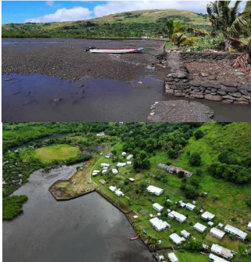
Figure 41: Project site at Nayavutoka Village
