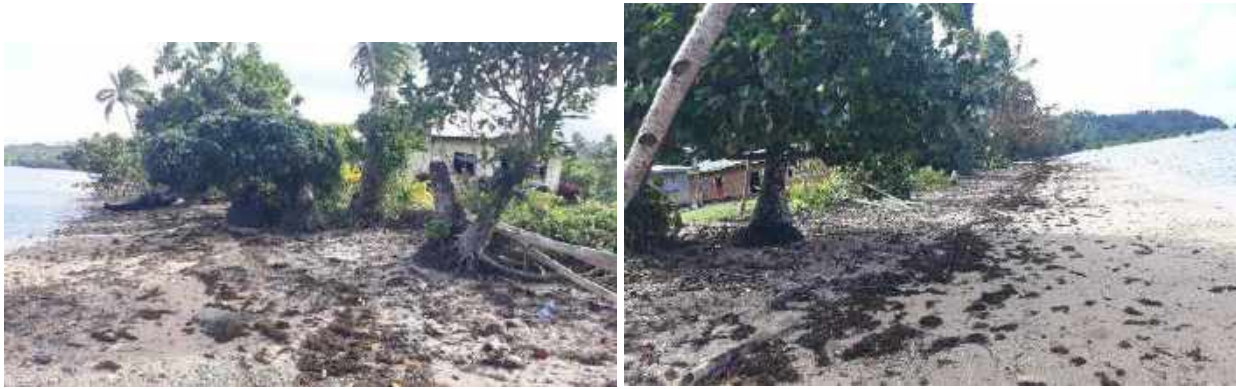
Figure 30: Project site at Saqani Village
