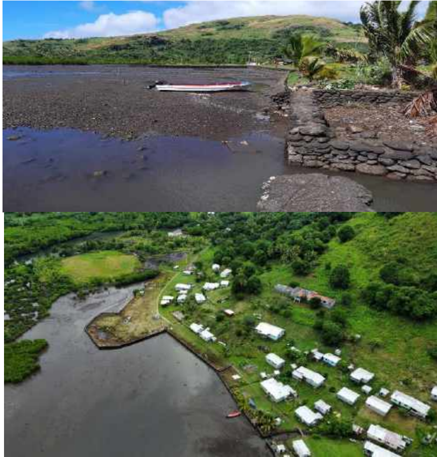
Figure 42: Project site at Nayavutoka Village
