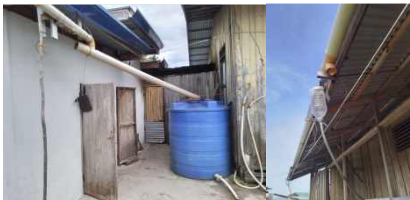
Figure 5. Existing rainwater harvesting systems, Sitangkai
