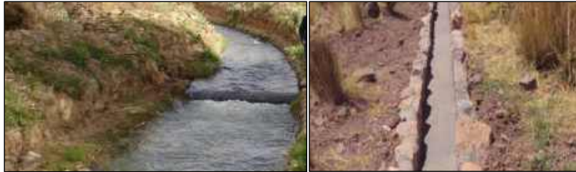
FIGURE 5. UNLINED IRRIGATION CANALS IN FIAMBALÁ, PROVINCE OF CATAMARCA. EXAMPLE OF A STONE-LINED CANAL, JUJUY PROVINCE
