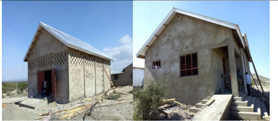
Food storage warehouse at Mairowa ward
