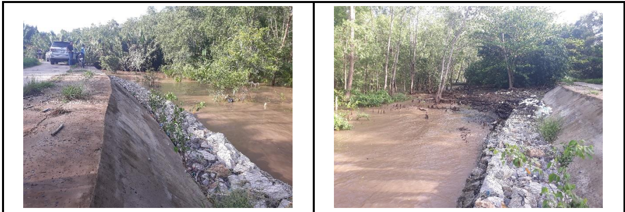
Figure 5.1 Installed concrete dike in Long Hoa commune
