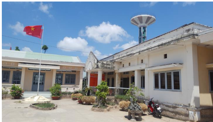
Figure 9. Water Treatment Plant in Hao Minh commune
