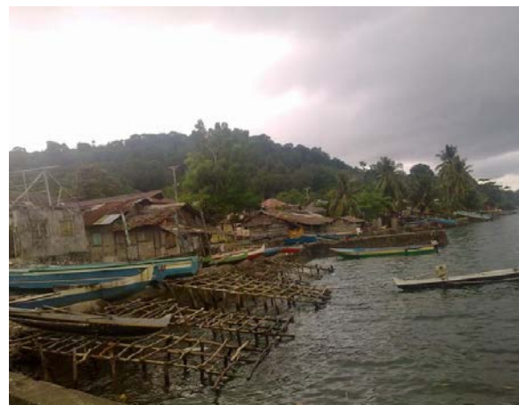
Figure 3. Fishermen built stilt structure for docking their boats due to the increase of sea water level
